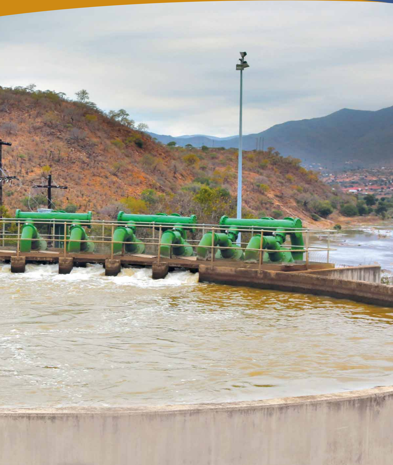
MADUNGELA PUMPSTATION PLANT
