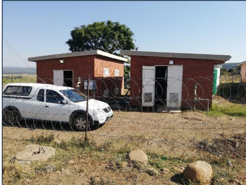
Figure 13.34 Khokwane Pump Station and Sahlumbe Pump Station on the Tugela Estates WTP site (Umgeni Water 2019).
