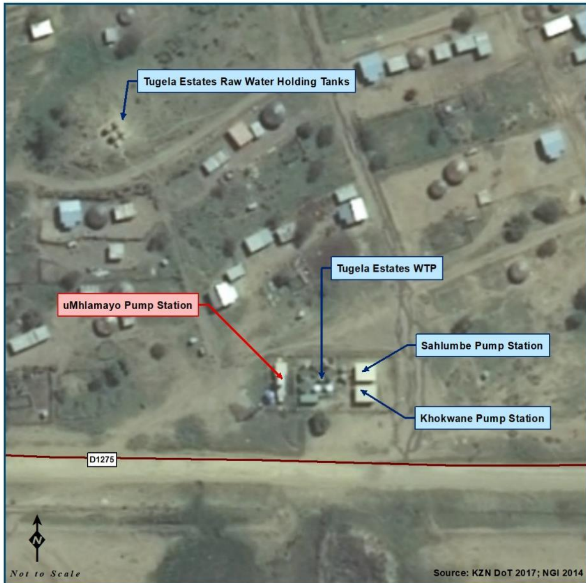
Figure 13.29 uMhlamayo Pump Station adjacent to the Tugela Estates WTP (KZN DoT 2017; NGI 2014).
