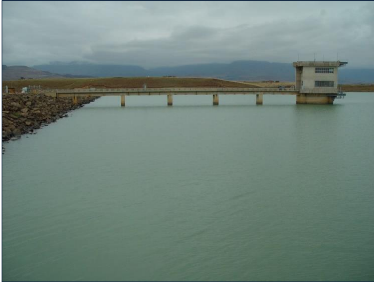
Figure 13.16 Woodstock Dam (DWS unknown date: DWS website).
