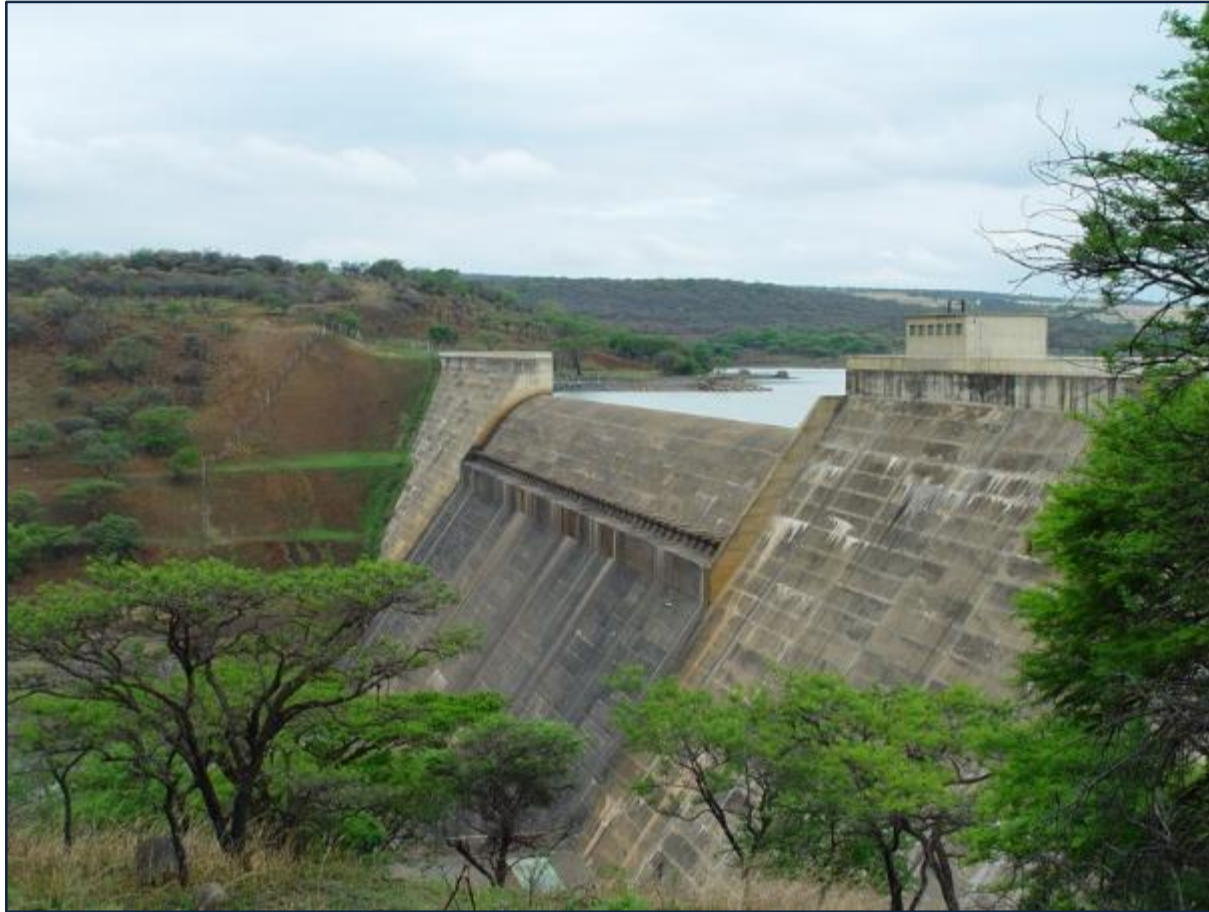
Figure 13.19 Spioenkop Dam (DWS unknown date: DWS website).
