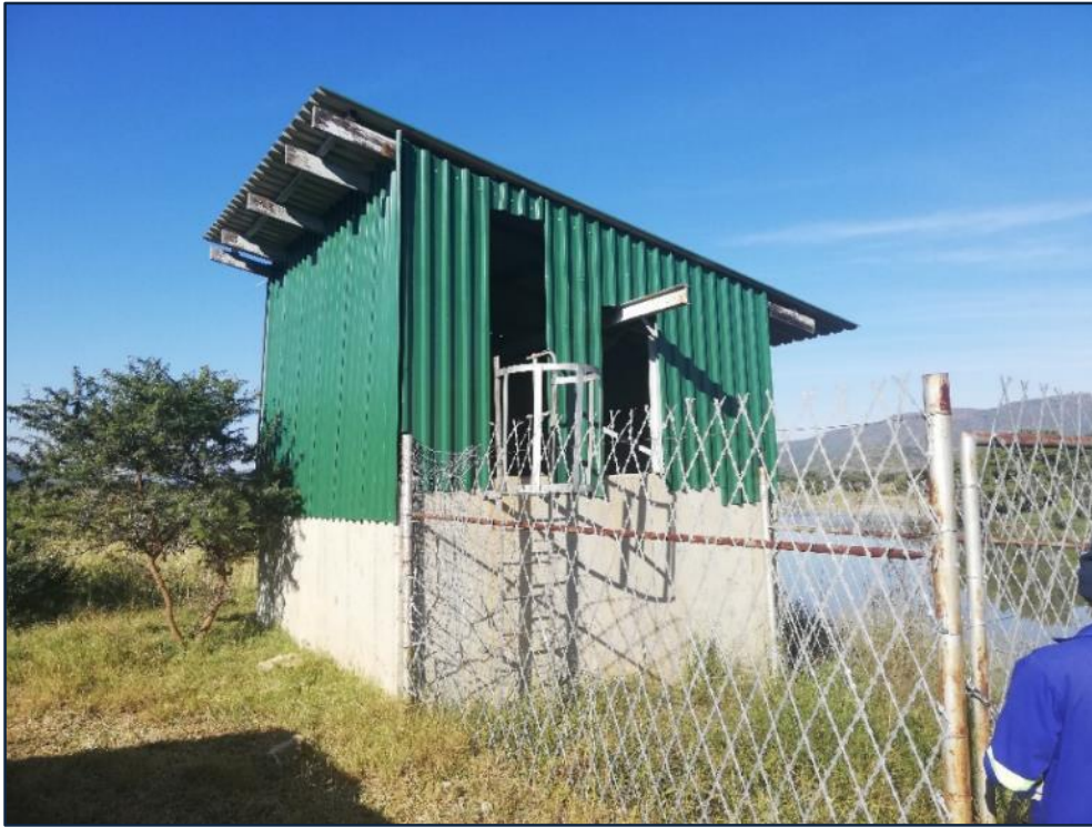
Figure 13.30 Tugela Estates Raw Water Pump Station (Umgeni Water 2019).
