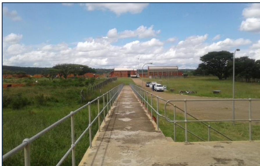
Figure 13.37 Olifantskop Water Treatment Plant (unknown date).
