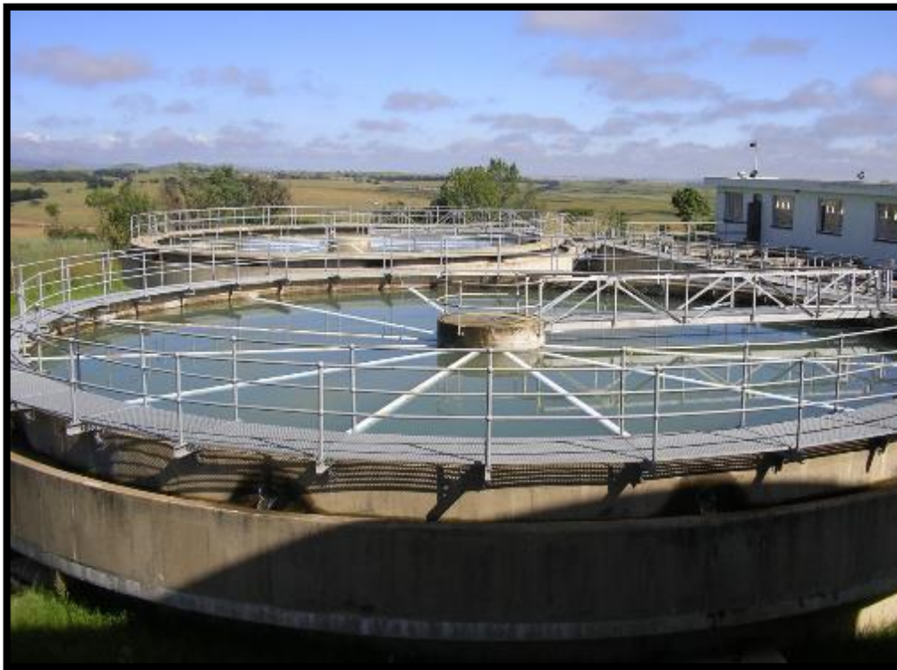
Figure 13.63 George Cross Water Treatment Plant (Bigen Africa, O & Manual, 2009)
