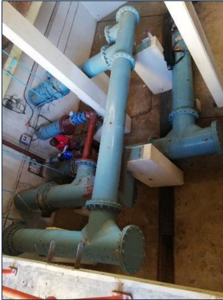
Figure 13.47 Waaihoek and Mabhekazi sales meters (Umgeni Water 2019).
