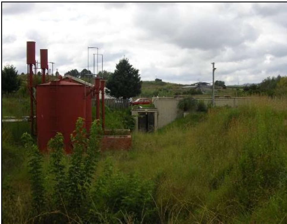
Figure 13.51 Bergville WTP (Bigen Africa, O & M Manual Bergville, 2009)
