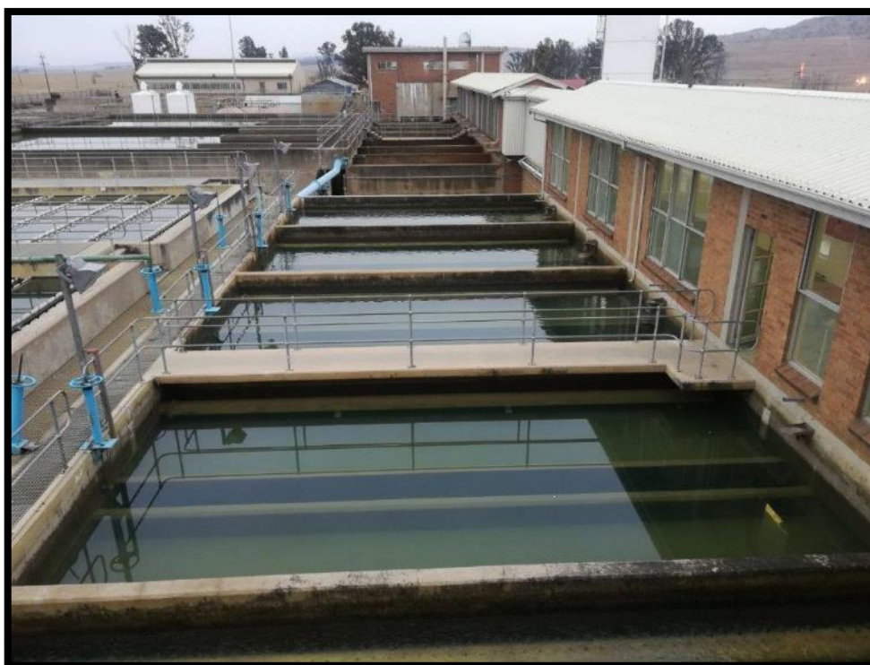
Figure 14.19 Photo of Ntshingwayo Dam (Primary Source of Ngagane WTP), May 2016
