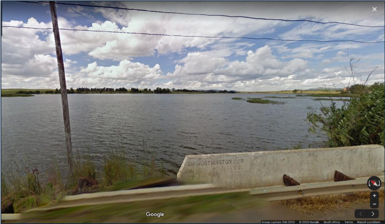
Figure 14.12 Tom Worthington Dam (Google StreetView 2010: website).
