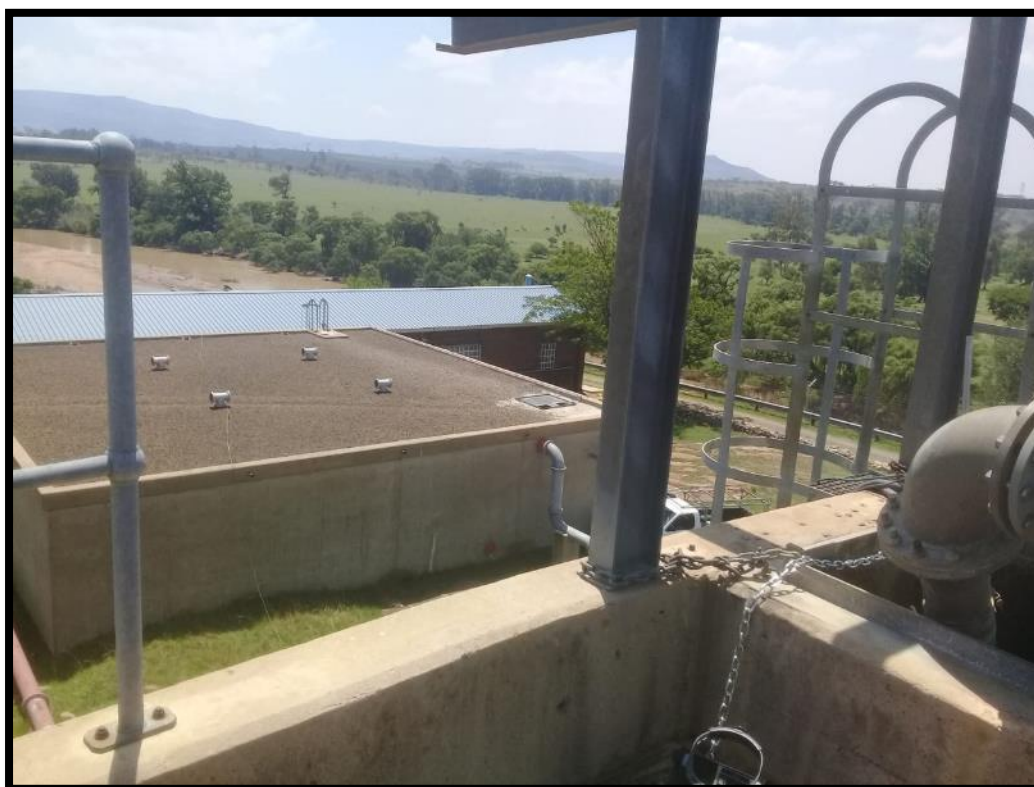
Figure 14.27 Photo of Vants Drift WTP (March 2020)
