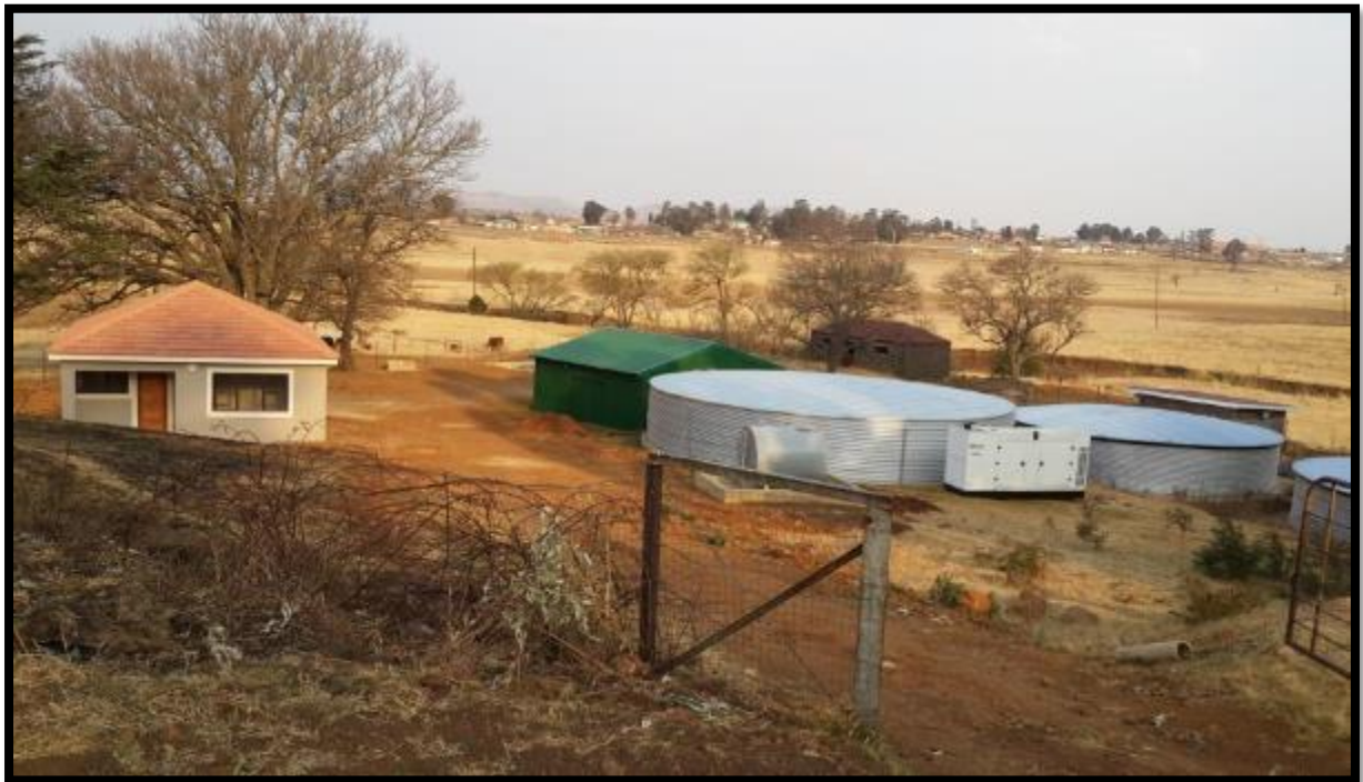
Figure 14.42 Photo of Charlestown Water Treatment Plant (July 2018).
