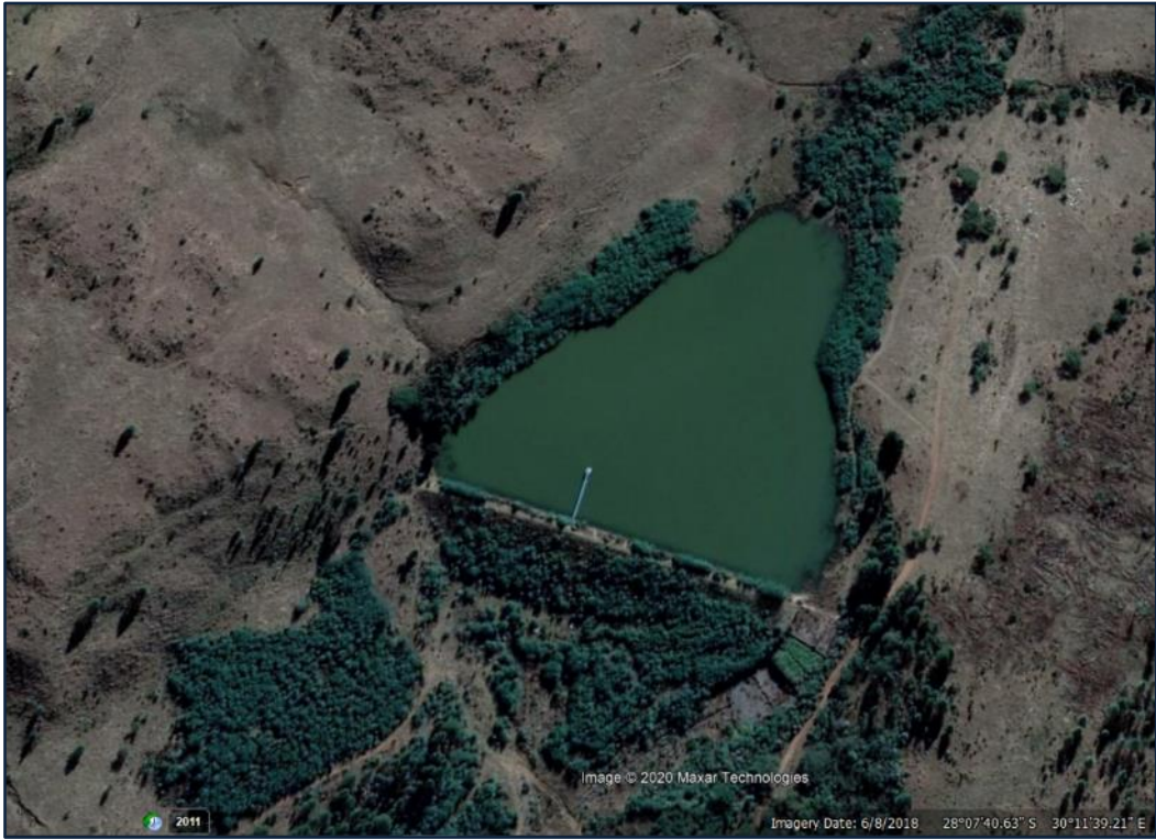
Figure 14.16 Upper Mpate Dam (Google Earth 2018: website).
