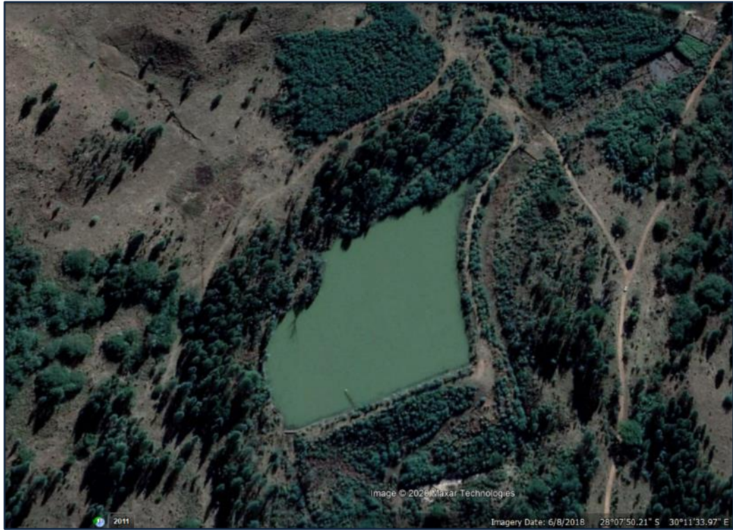
Figure 14.17 Lower Mpate Dam (Google Earth 2018: website).
