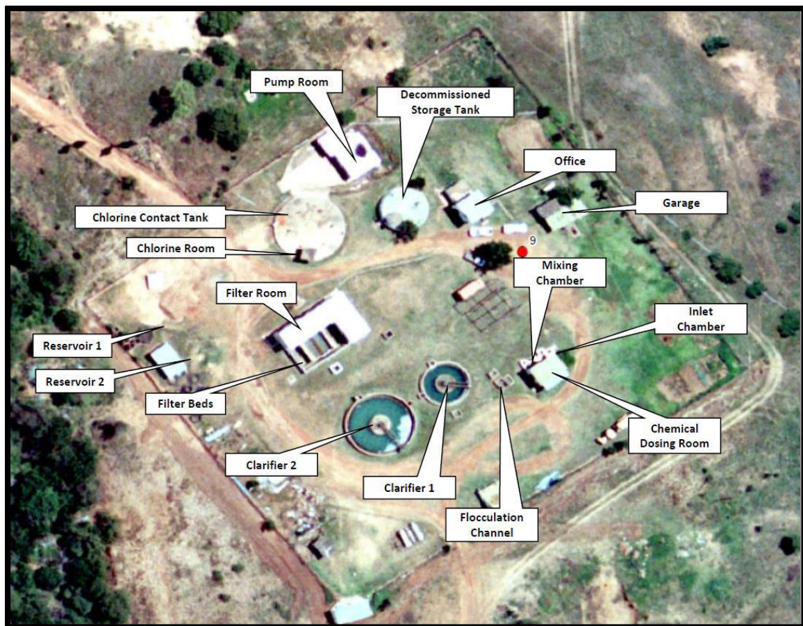
Figure 14.37 Aerial Image of Utrecht Water Treatment Plant (ADM O&M Manual May 2016)
