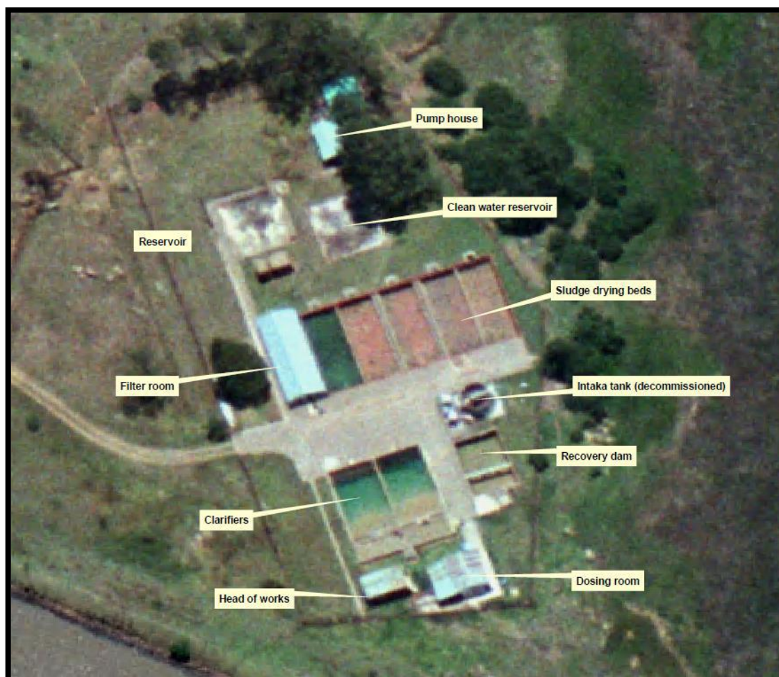
Figure 14.30 Aerial Image of Dannhauser Water Treatment Plant (ADM O&M Manual May 2016)
