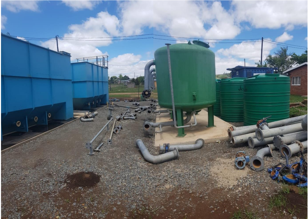
Figure 7.76 1 MI/day being constructed at the Lidgetton System.
