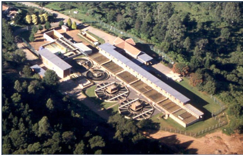
Figure 7.35 D.V. Harris Water Treatment Plant.
