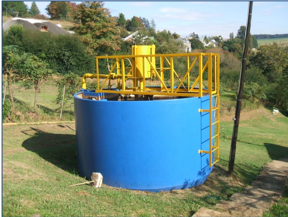
Figure 7.84 Rosetta WTP (uMgungundlovu District Municipality 2010).
