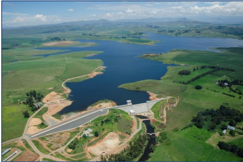
Figure 7.26 Spring Grove Dam.
