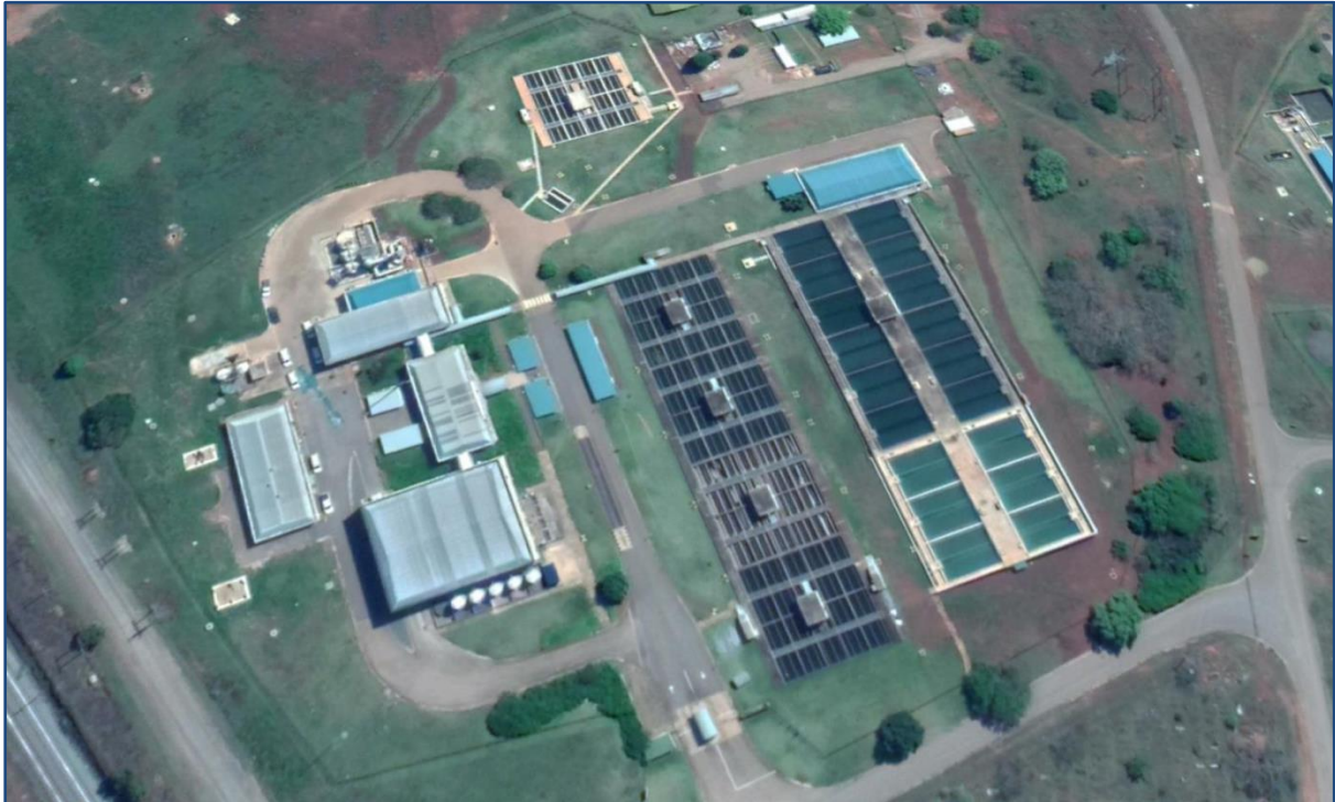
Figure 7.29 Midmar Water Treatment Plant after the upgrade.
