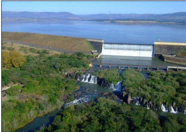
Figure 7.22 Albert Falls Dam.
