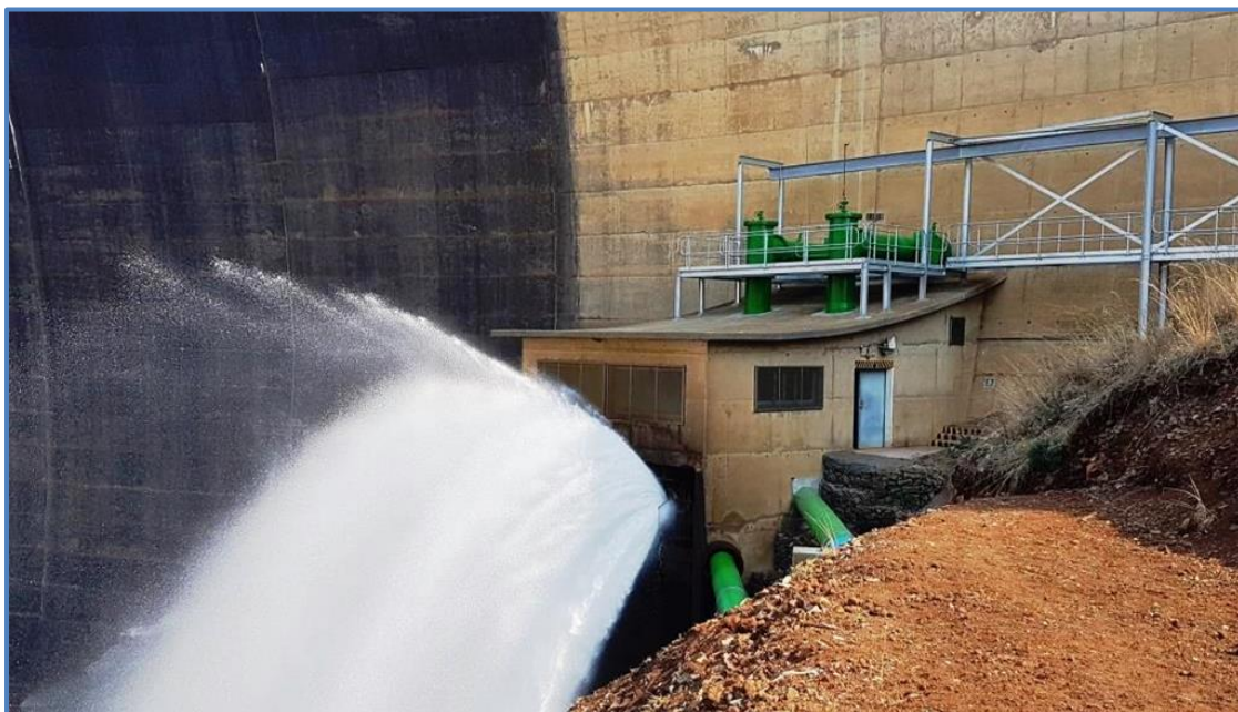
Figure 12.47 Abstraction point (Craigie Burn Dam)
