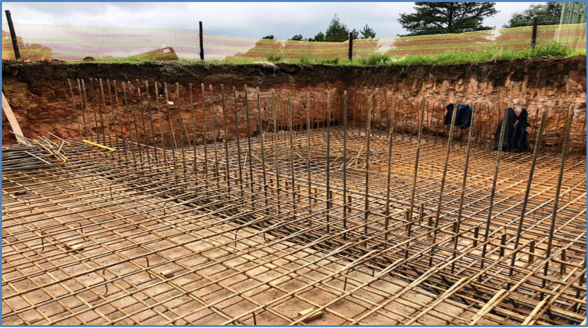
Figure.12.48 Transfer Pump Station in Construction (Late 2019)
