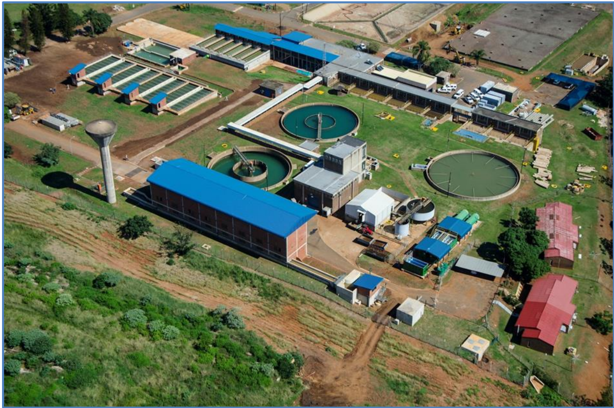
Figure 12.18 Hazelmere Water Treatment Plant.
