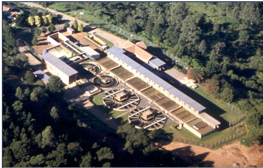
Figure 7.38 D.V. Harris Water Treatment Plant.
