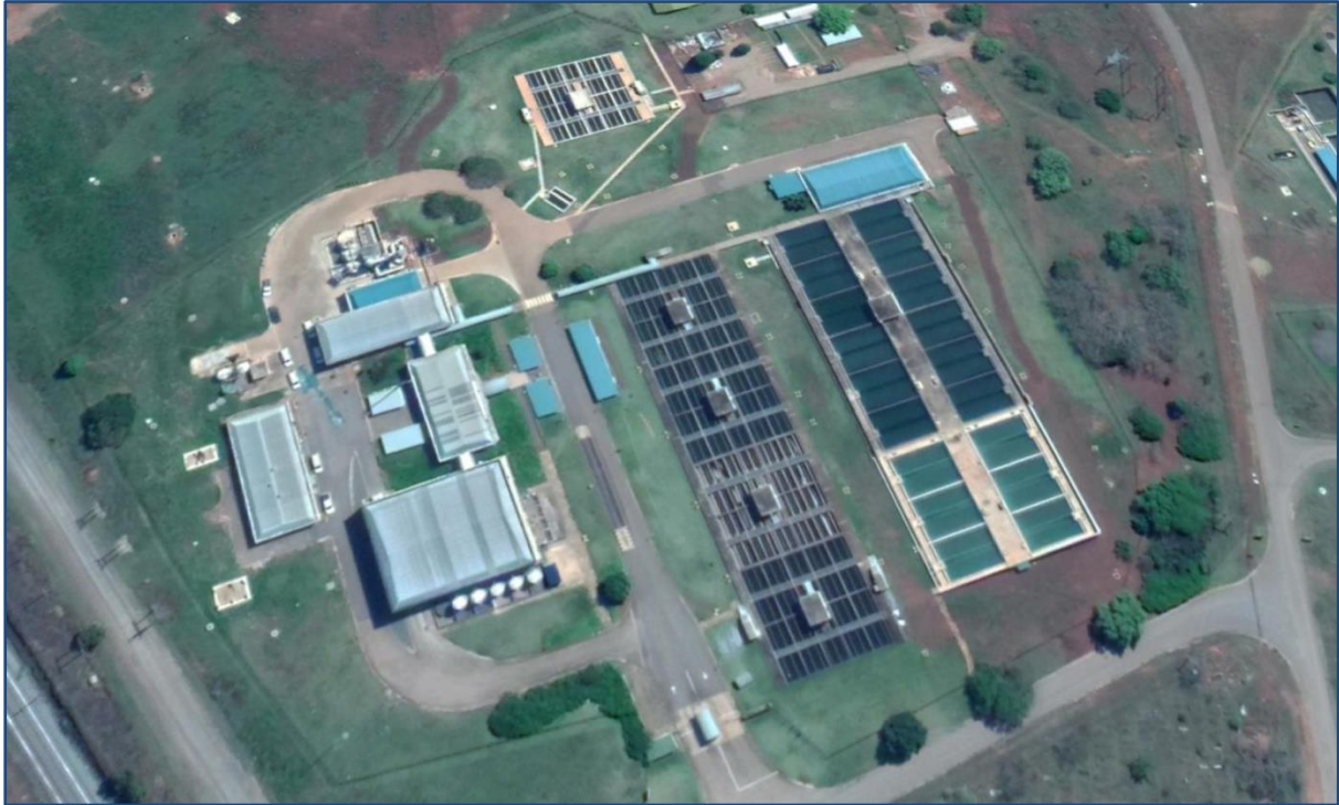
Figure 7.32 Midmar Water Treatment Plant after the upgrade.
