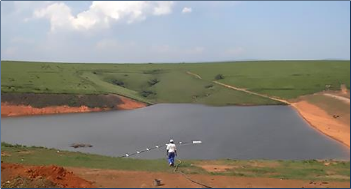
Figure 15.4 Ntingwe Dam (MBB Consulting Engineers 2020: website).
