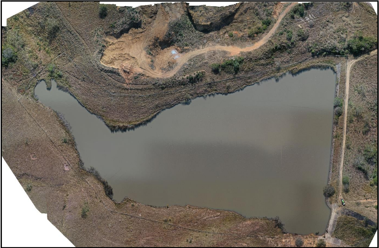
Figure 16.5 Melmoth Off-Channel Storage Dam (UW, 2022).
