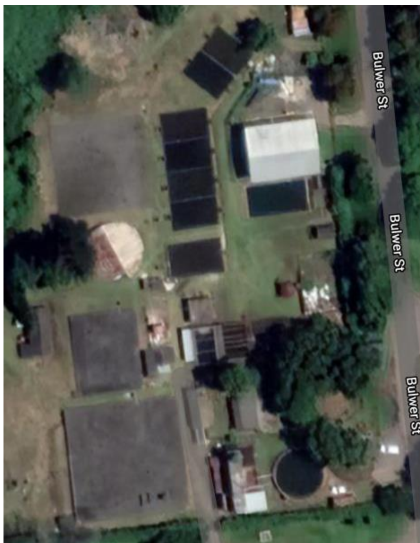
Figure 16.22 The Eshowe WTP.
