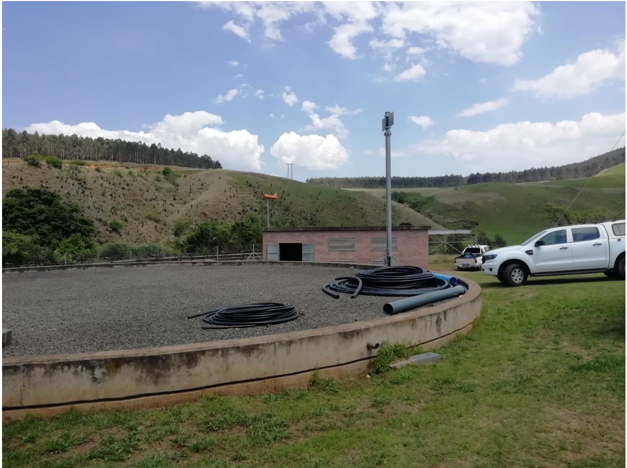
Figure 16.12: The Nkandla WTP (Photo taken by UW).
