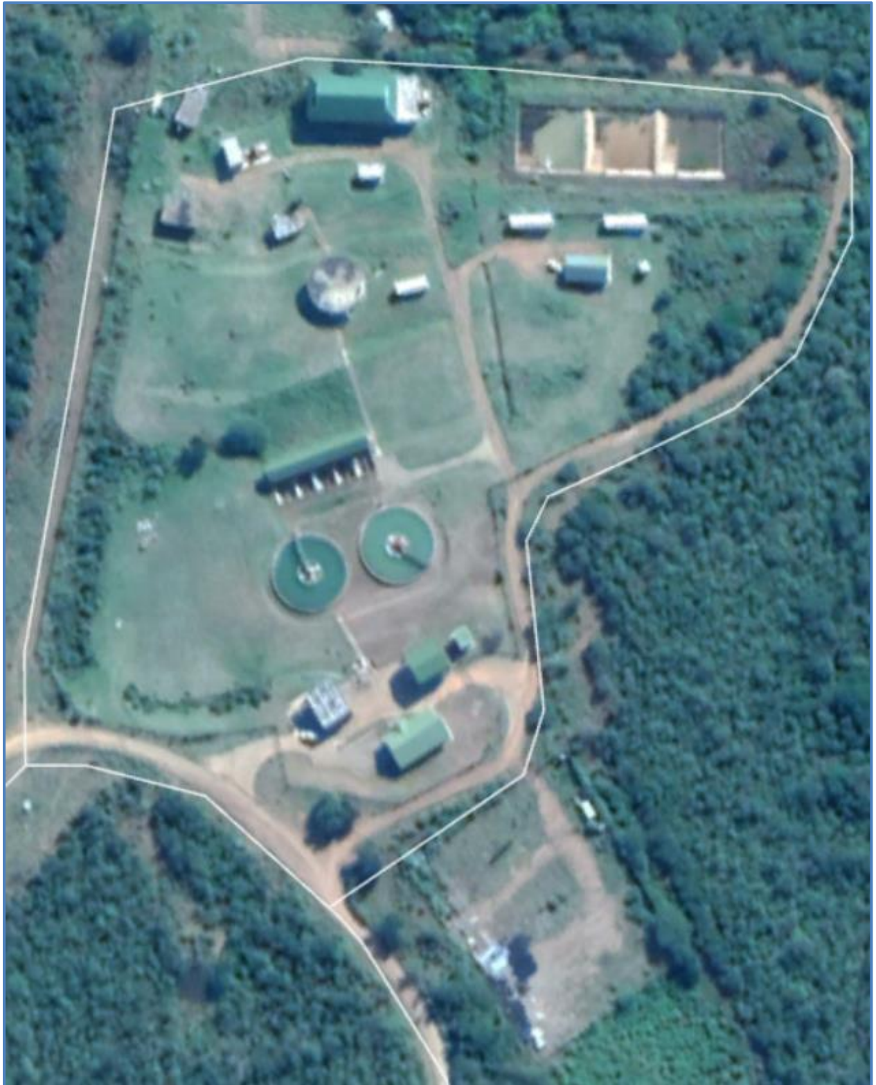
Figure 16.20 Greater Mthonjaneni WTP.
